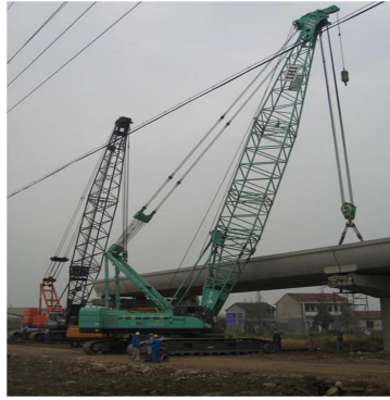
Figure 1: Placing full precast span (with crane)
