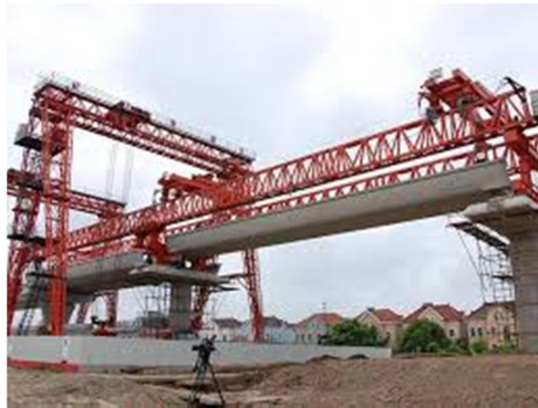
Figure 2: Placing full precast span (with launching girder)
