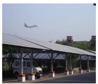
Minimum height and width for elevated structure of service structure shall be 5.5 m Minimum height for parking structure of service structure shall be 2.5 m
